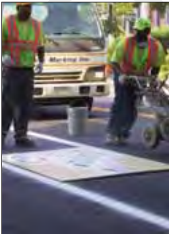
Bike lane installation, New Haven
