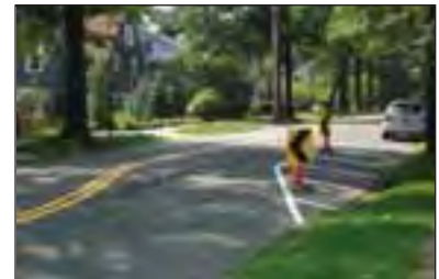
Chicane on Vista Terrace, New Haven
