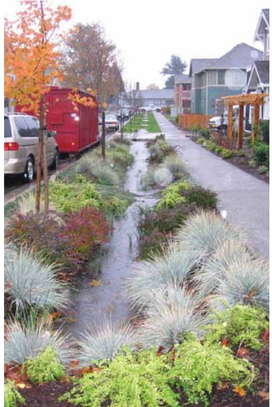
Bioswales used to capture and maintain runoff water
