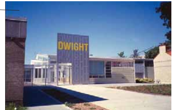
Dwight School Addition
