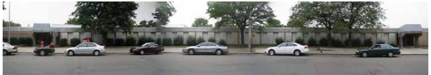
Current Dwight School facade
