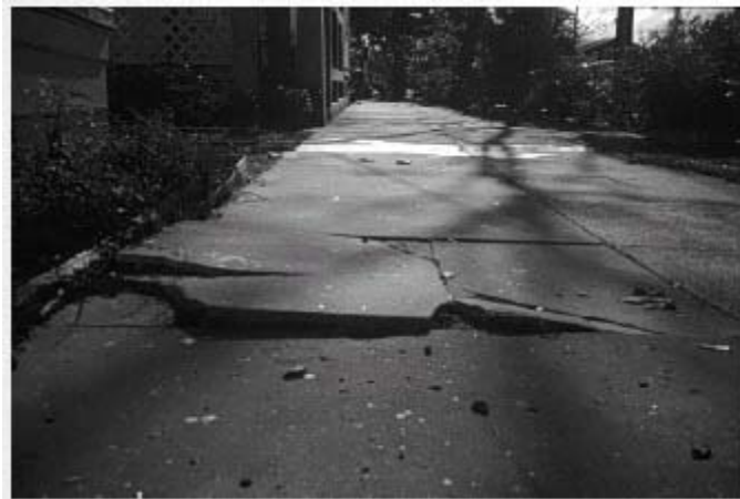
Figure 10-1. Regular sidewalk maintenance can prevent or correct sidewalk conditions, such as changes in level.
