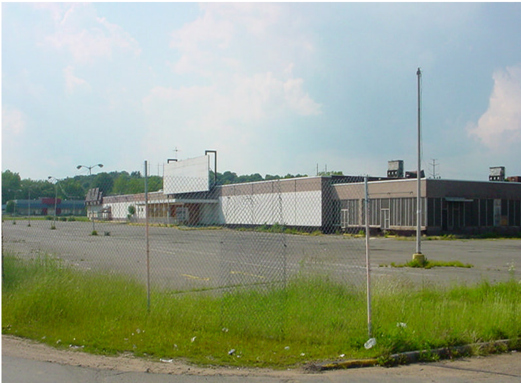
Abandoned "big box" stores are good sites for productive re-use.
